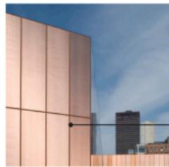
*okalux or similar glazing solution to customize and control the level of transparency of the training room glazing*
