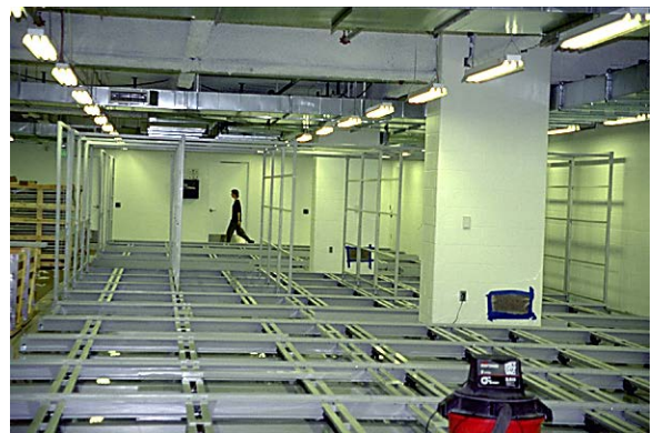
Compactor Carriages Installed in New Vault
