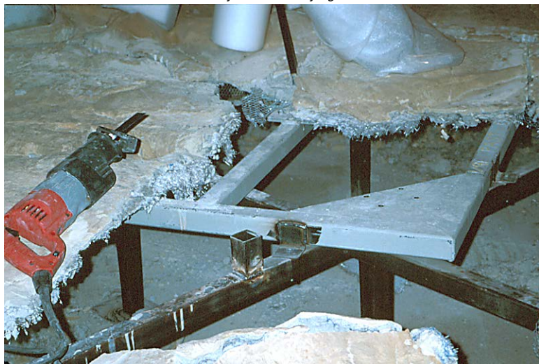
Metal Mesh "Rock" of the Old Museum's Dinosaur Display is cut away from underlying steel.
